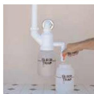
The water in the upper portion of the trap will drain down....
