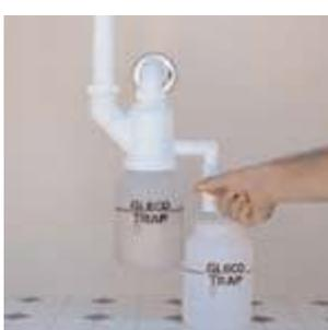
Place the new, empty bottle under the valve and open
